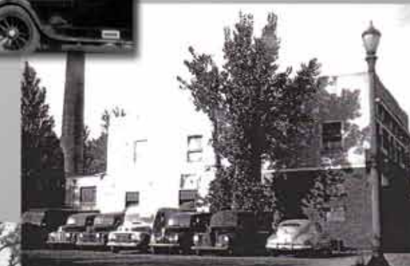
Industrial Service Company
